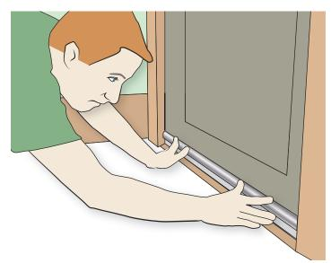
**Older doors and windows** are more difficult to airseal. Most have single pane windows held in place with putty and insuring they are properly secured is the first step. There are various types of weatherizing and airsealing materials that can be creatively used including adhesive backed foam, metal or plastic v-seal, rubber bulb type, etc...
